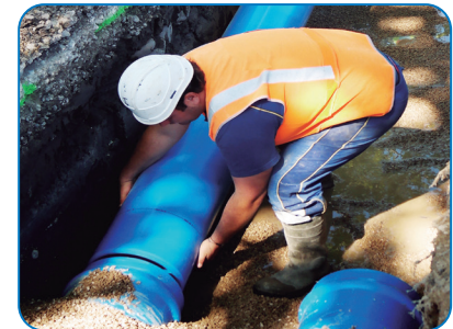
The length limit mark for the assembly of the pipes is the distance from the beveled end of the pipe to the printed cutting mark.
